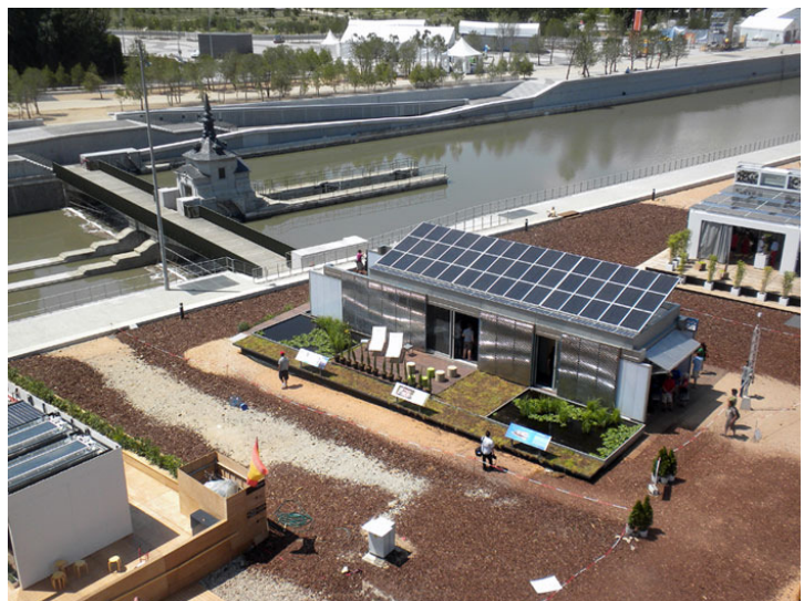
The Virginia Tech Lumenhaus at the 2010 Solar Decathlon Europe
